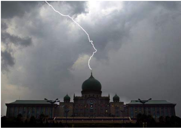
Fig. 8: A photograph of lightning striking the ESE air terminal on the Prime Minister Department building. (Photo credit: The Star Publications plc)
