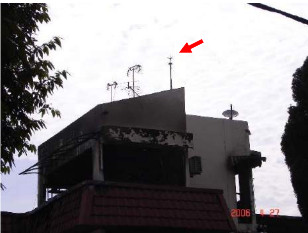
Fig. 4: Close-up view of the ESE air terminal on the roof (arrowed).
