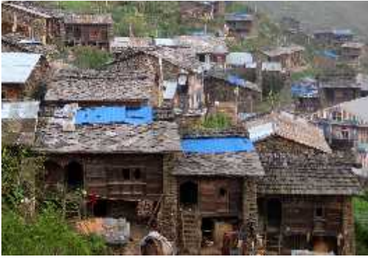
Figure 12: Typical attached Tamang house with elevated ground floor
