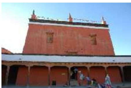
Figure 16: Typical Small windows in building façade in Upper Mustang
