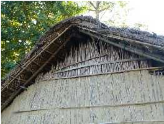
Figure 7: Gable opening for air circulation in Tharu House, Chitwan
