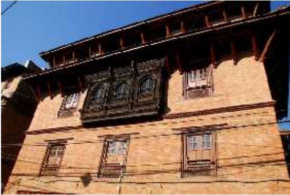
Figure 10: Façade of Newar house with big wood carved window and large roof overhang
