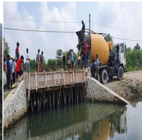
Culvert Casting at (NCB-03)
