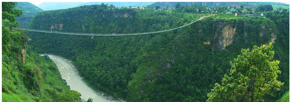
Bangechaur-Aaduwabari Bridge (Baglung-Parbat), -Longest Suspension Bridge (span :- 567m long)
