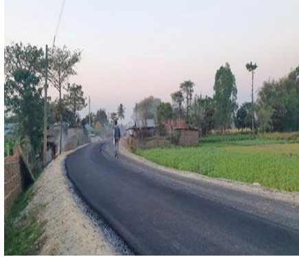
Asphalt Work, Sunsari(NCB-03)
