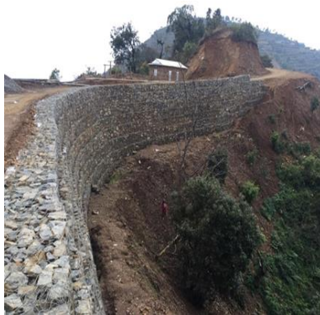
Gabion Work, Chitwan (NCB-09)
