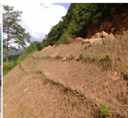
Bio-engineering works in Road-1 (NCB-10)
