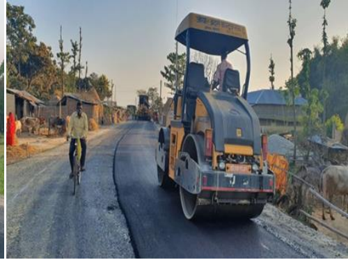
Asphalt Laying, Sunsari(NCB-03)
