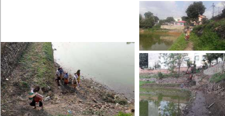
First phase work – clearing debris of the lowest level
