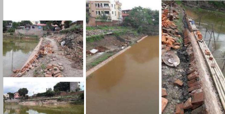
First phase work – Repairing the lowest level inclined wall
