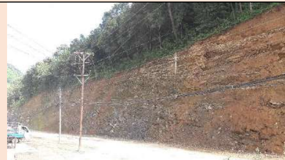
(b) Road widening in Waling municipality
