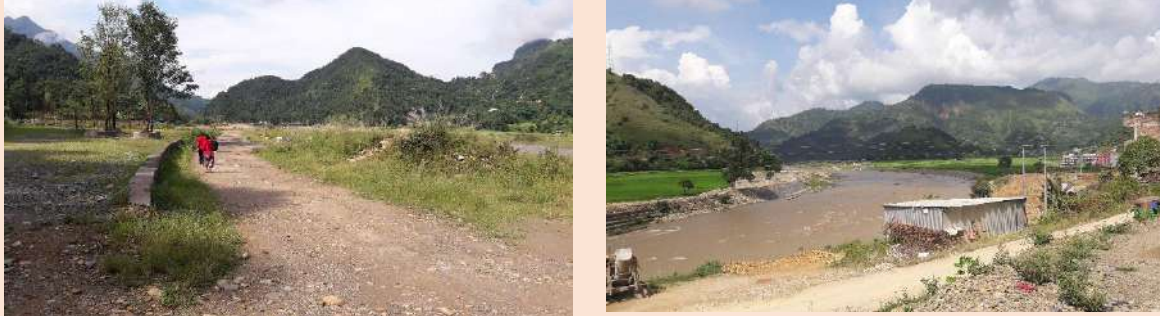
(a) Construction of road on both sides of river in Putalibazar
