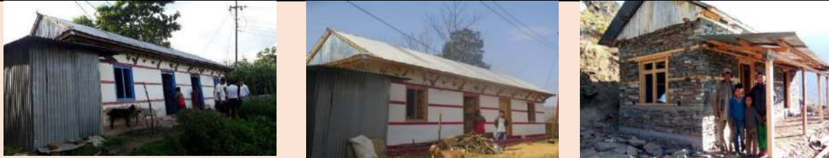
Demonstration houses for most vulnerable families in Dolakha, Sindhupalchowk and Kavrepalanchowk
