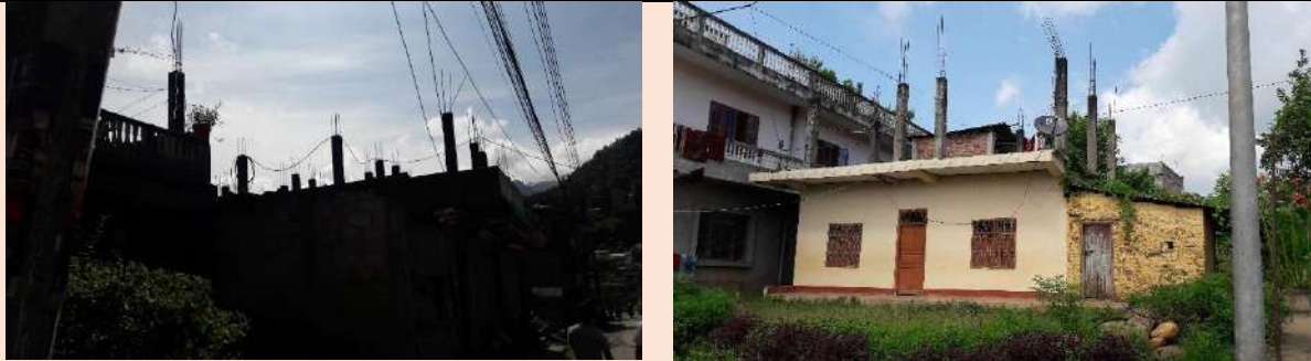
(a) Exposure of iron rods for future expansion in Putalibazar
