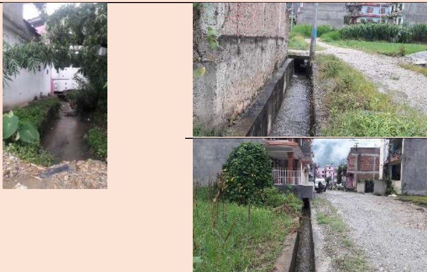
Fig. 12 Encroachment of drainage
